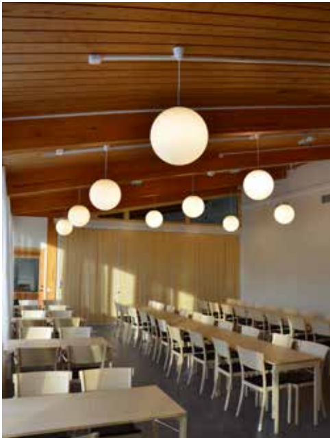
Church in Bollnora, Sweden. Wooden ceilings treated with ES/VFR flame retardant coating to B s1 d0.
