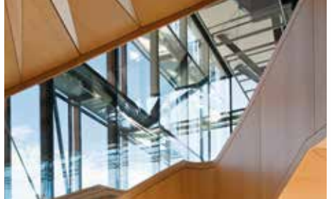
Concert Hall in Stavanger, Norway. Interior wood veneer and MDF treated with ES/VFR flame retardant coating to B s1 d0
