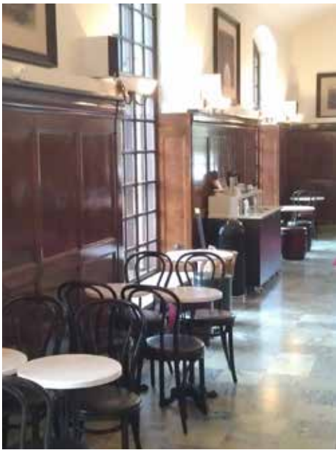
Starbucks in Malmö, Sweden. Wood paneling treated with ES/VFR flame retardant coating to B s1 d0.
