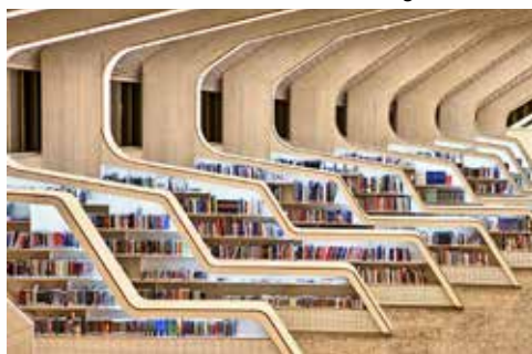
Vennesla Library in Norway. Interior supportive glulam beam system treated with ES/VFR flame retardant coating to B s1 d0.
