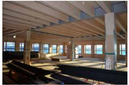
Kongsvinger Festing in Norway. Internal wood treated with HW01 intumescent paint to EI30.
