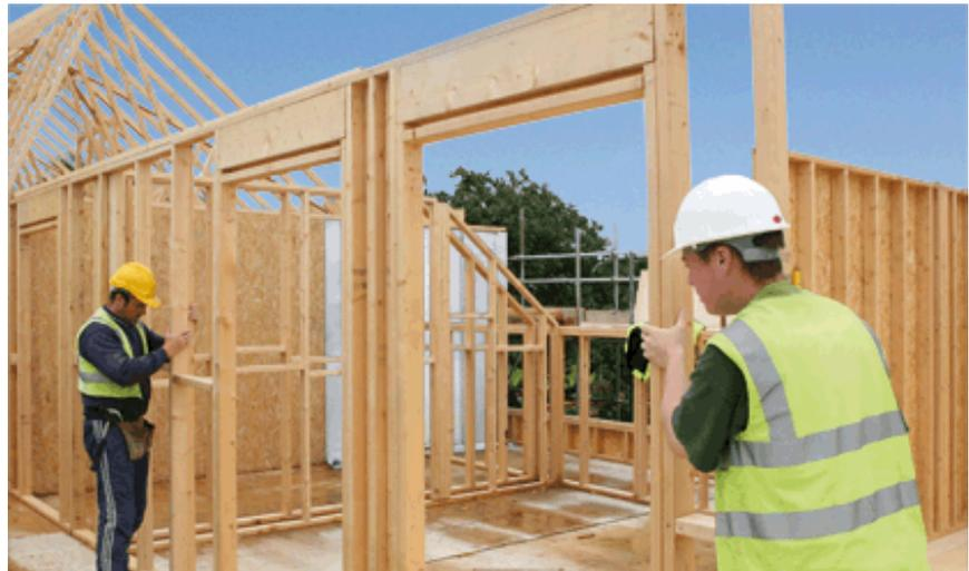
Figure 2: Installing open panels. Photo: Castleoak Group
