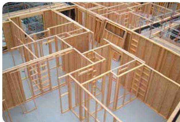
**Figure 1:** Modern timber frame construction
