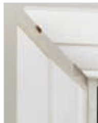
9. Fit and Fix architraves in place
