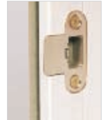
4. Keep is provided fixed to the lining
