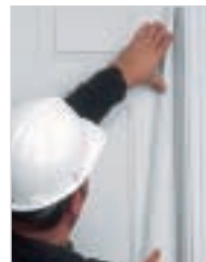
10. Fit and Fix door stops in place
