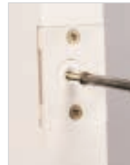
7. Remove 'grommit' in door hinge which allows frame hinge to locate. Reposition 'grommit' when in place
