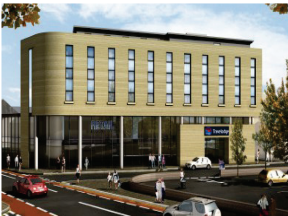
Kempston Travelodge, Lancaster Timber Frame Contractor - Shire Timber Structures Main Contractor - Sisk UK Ltd Image - Sisk UK Ltd
