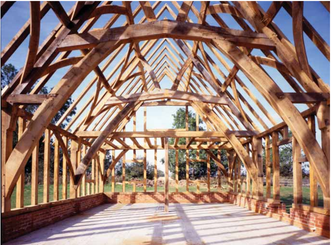
Figure 2.10 (and next page) Modern green oak structures Framing and photos: The Green Oak Carpentry Company below: Completed frame before enclosure
