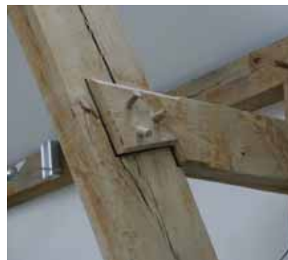
Figure 1.3 The natural fissures which develop in a green oak frame as the timber dries. Photo: Ian MacNicol
