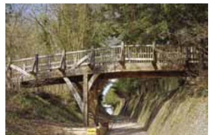
9.11 Polesden Lacey bridge
