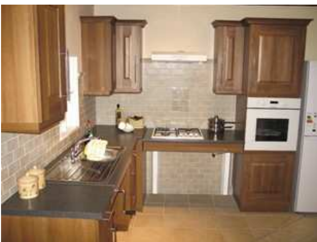
Kitchen units designed for use by wheelchair users. Future adaptations such as those shown above should be relatively easy to make when required.
