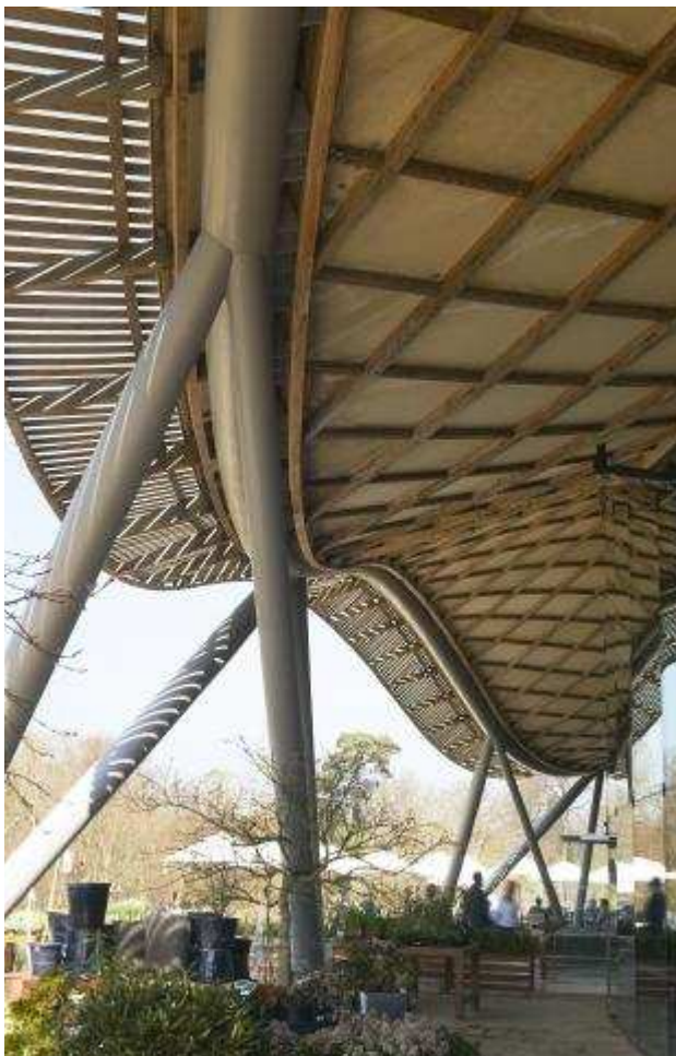
Fig 1 Saville Building, Windsor Great Park - designed using Eurocode 5: External decking
