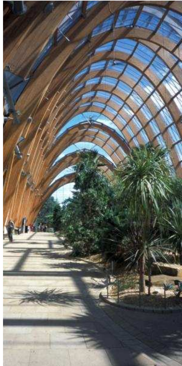
Fig 7 Sheffield Winter Gardens, courtesy of Buro Happold, Structural Engineers: Internal view
