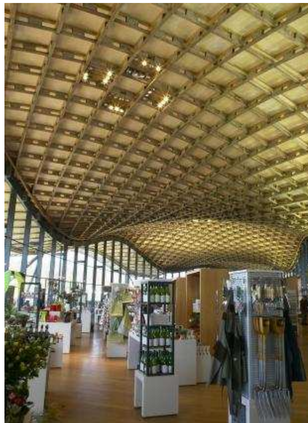
Fig 6 Saville Building, Windsor Great Park: Underside of roof in gift shop
