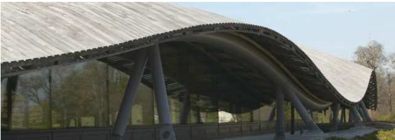
Fig 5 Saville Building, Windsor Great Park: External roofline
