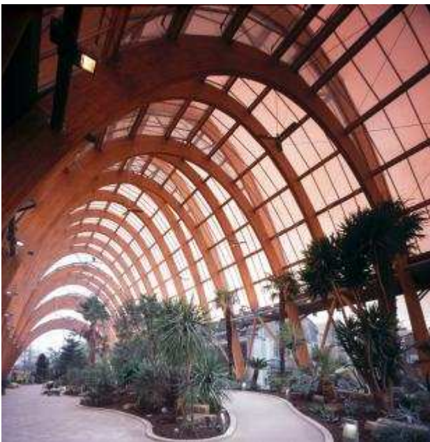
Fig 2 Sheffield Winter Gardens, courtesy of Buro Happold, Structural Engineers: Internal view
