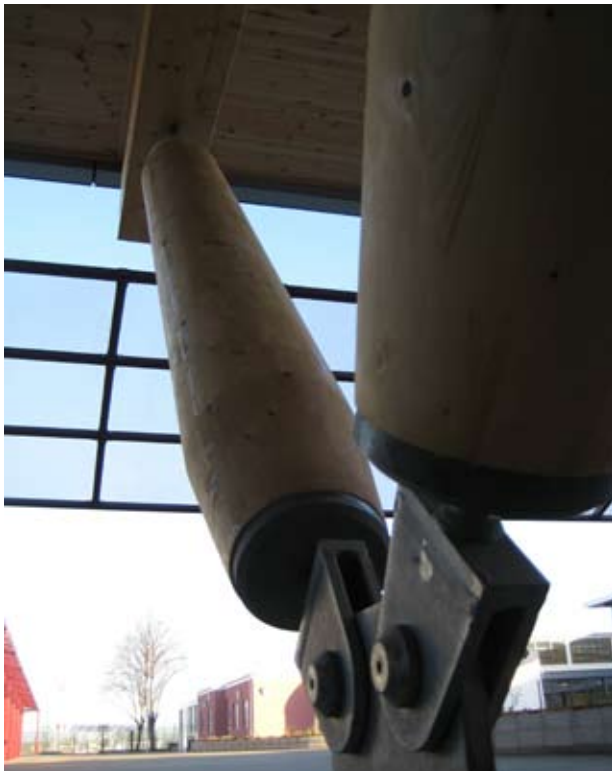
Fig 2. Glulam columns at St John Fisher School in Peterborough, Cambridgeshire, designed with EC5. Photo courtesy of Ramboll UK.
